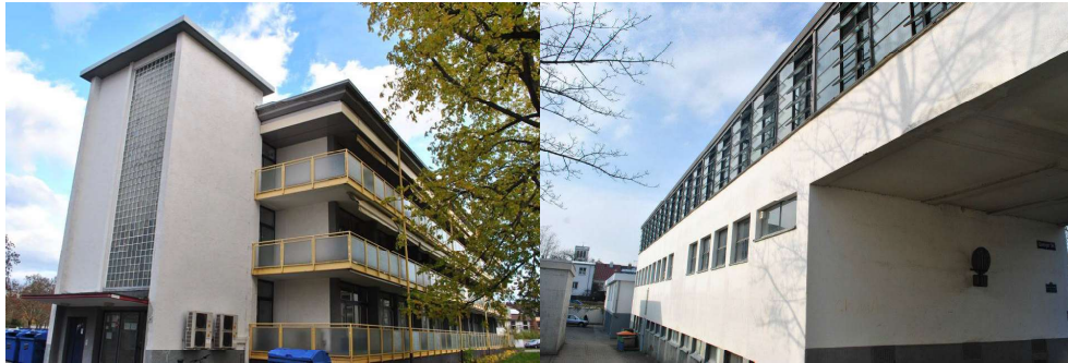
Figures 2a and 2b: Schwesterwohnheim, Today Kolleg am Ring of Wohnheim e.V. of the Karlsruhe Institute of Technology, Architects Otto Haupt, Heinrich Müller, (1951), Current State and Former Washing Salon of the Dammerstock Siedlung in Karlsruhe, Architect Otto Haesler (1929)
