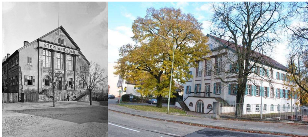
Figures 3a and 3b: Stephaniensbad in Karlsruhe, Architect Friedrich Weinbrenner (1811)
